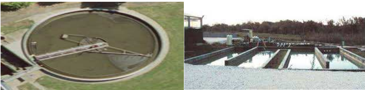
Fig 1: Types of Sedimentation tank
